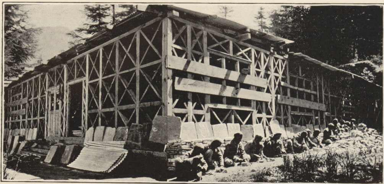
THE EARTHQUAKE PROOF DHAJJI DIWAR CONSTRUCTION.
